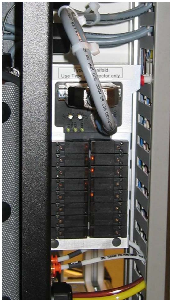
Figure 46. Valve manifold which is mounted on the outside of the gas box towards the front of the system.
