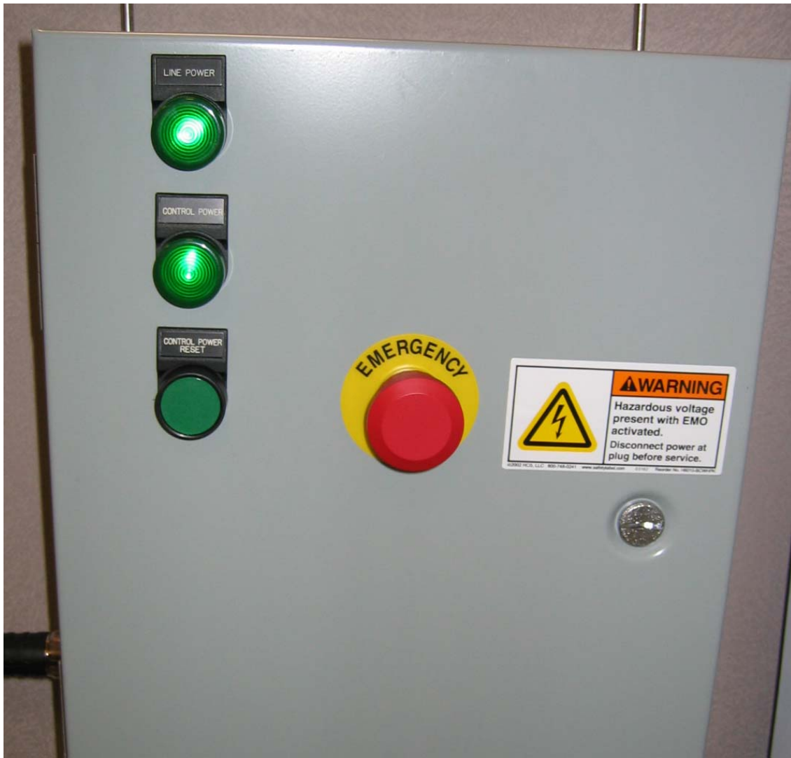
Figure 25. Power control box with indicators and control power reset.
